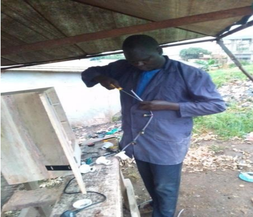
Figure 8 showing the connection of bulb holders
